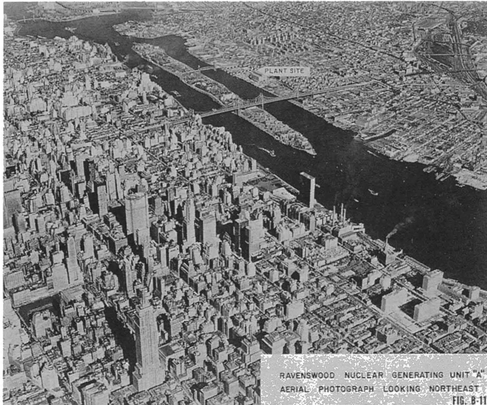
4. Site of proposed Ravenswood nuclear plant in New York City. The Empire State Building is at the lower left; the United Nations is in the center along the East River. (AEC Docket 50-204)
