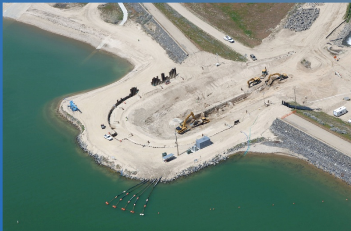
Deer Flat Dam Interim Repair Upstream Berm
