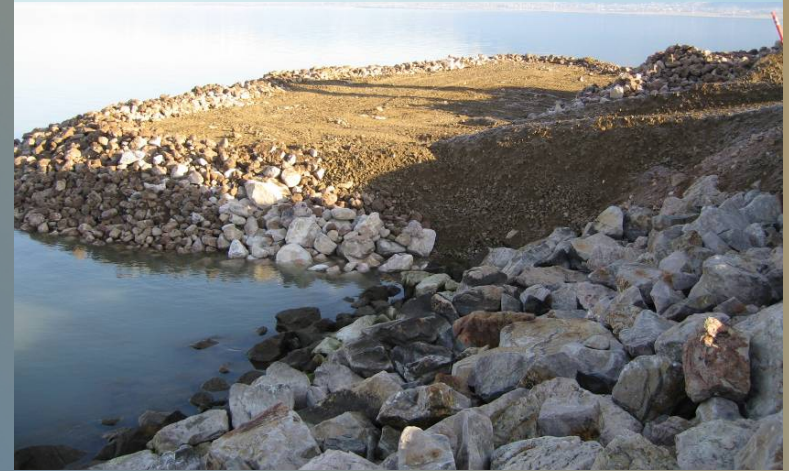
A.V. Watkins Dam Emergency Repair Upstream Berm
