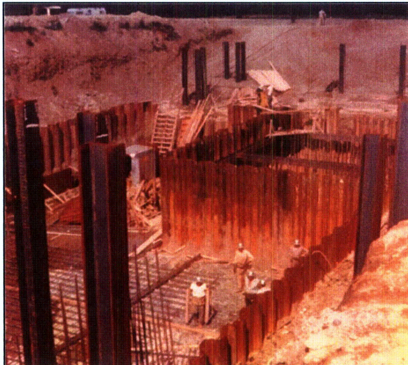
Figure 4C2-1. Construction Photograph Showing Foundation Pilings 36 8/14/09
