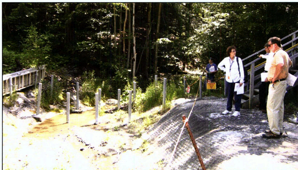
Figure 5C11-1. Franks Creek Looking Upstream
